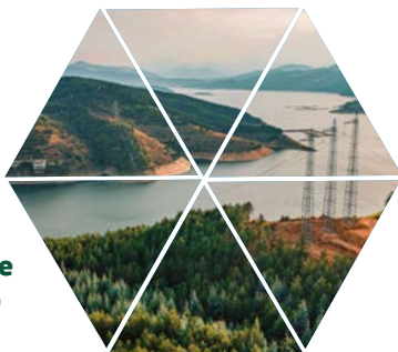
Electricity line between Maritsa East and Nea Santa near the municipality of Haskovo, BG
